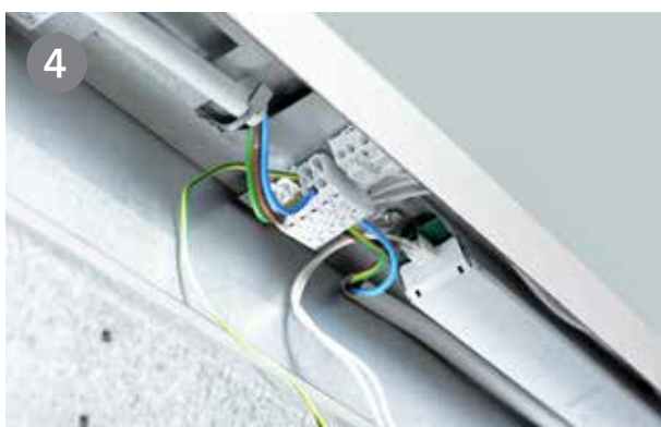
4 Connect the cable to a through-wiring 5-way terminal block.
