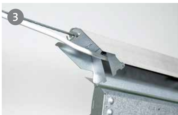
3 Place the cable through a slotted opening in the outer end-cap and secure it with the cable rack.
